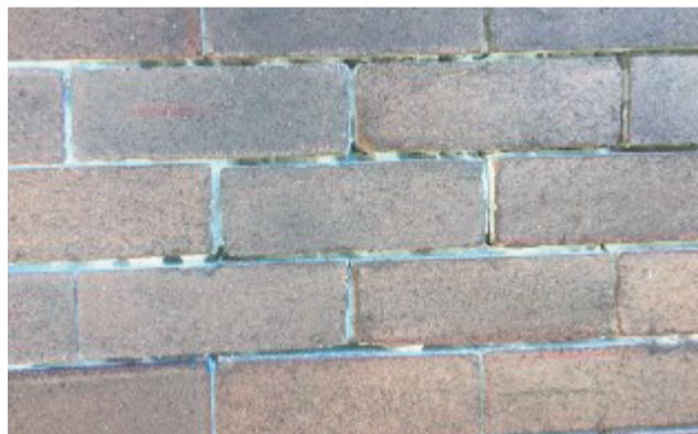
The holes created by the mortar bee are evident in the mortar.
